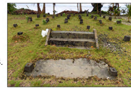
Photo E. Remains of Iroiijlaplap Litokwa's Residence
